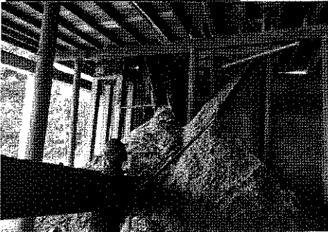
Area under wet sawmill:
